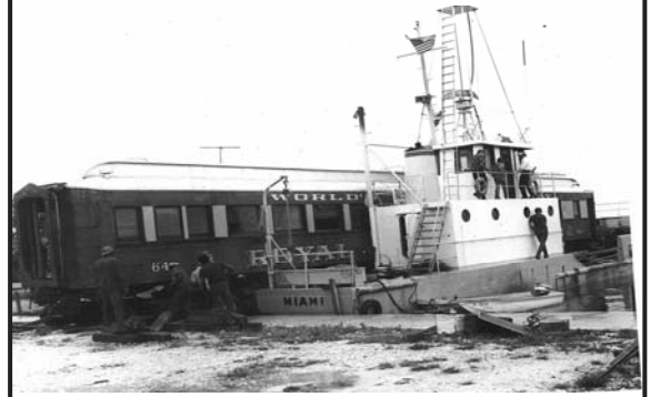
The Florida East Coast Railway car being barged into Knights Key where it can be seen today.
